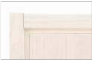
VISTA INTERNA INTERNAL VIEW
